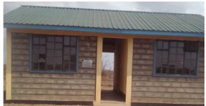
Above, new administration office and staff room at Kachiuru
