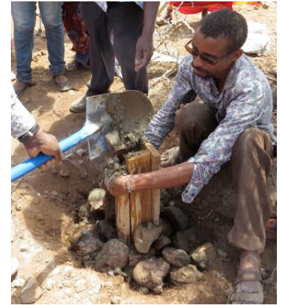
Filling the marker form with concrete
