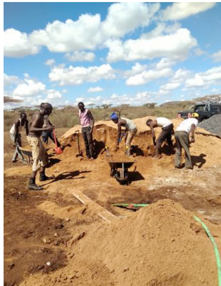
Excavation work on the cattle dip
